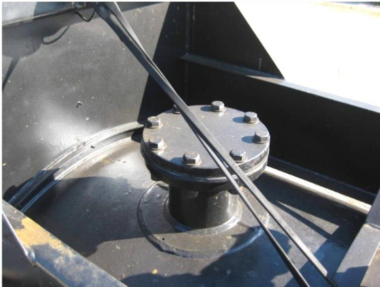
**Figure F10 - Torqued bolts not protected**
