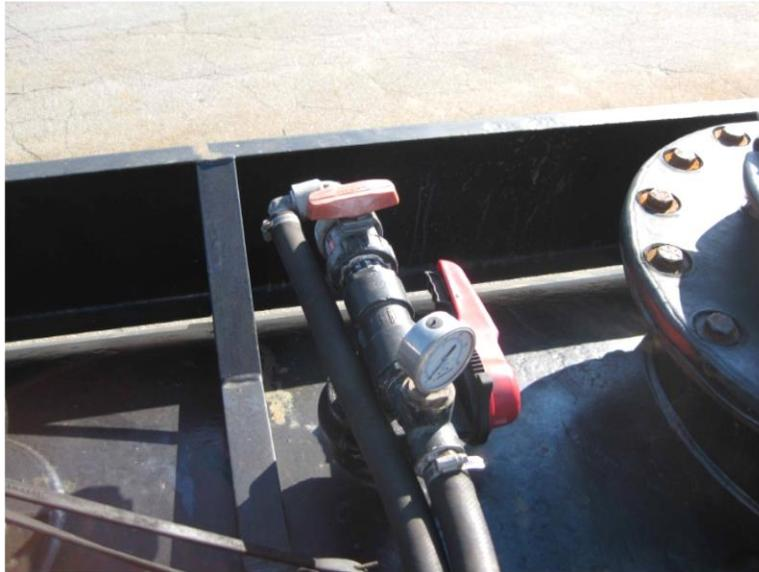
**Figure F9- Miscellaneous in-line plumbing not protected**
